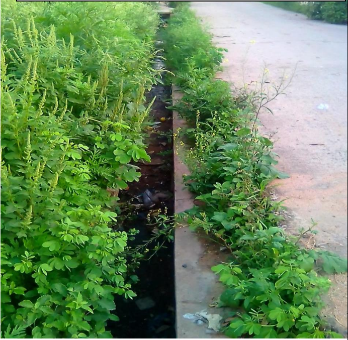
BEFORE W.NO.22, ESHWAR NAGAR BACK SIDE
